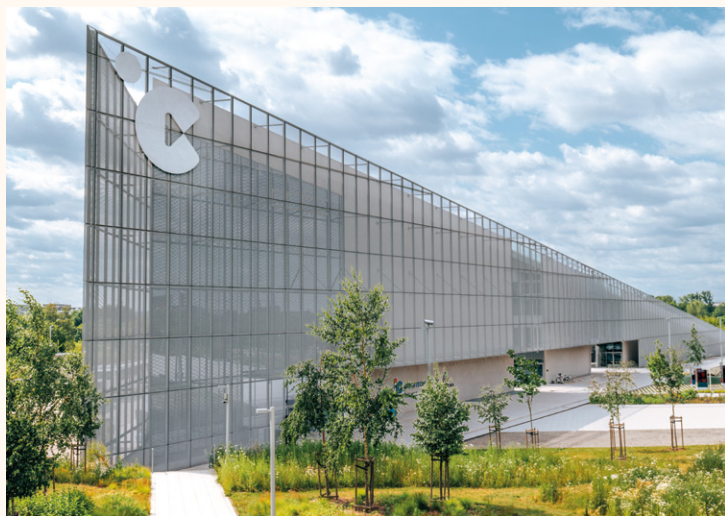
The award-winning Cogiteon building | photo: MCN Cogiteon
